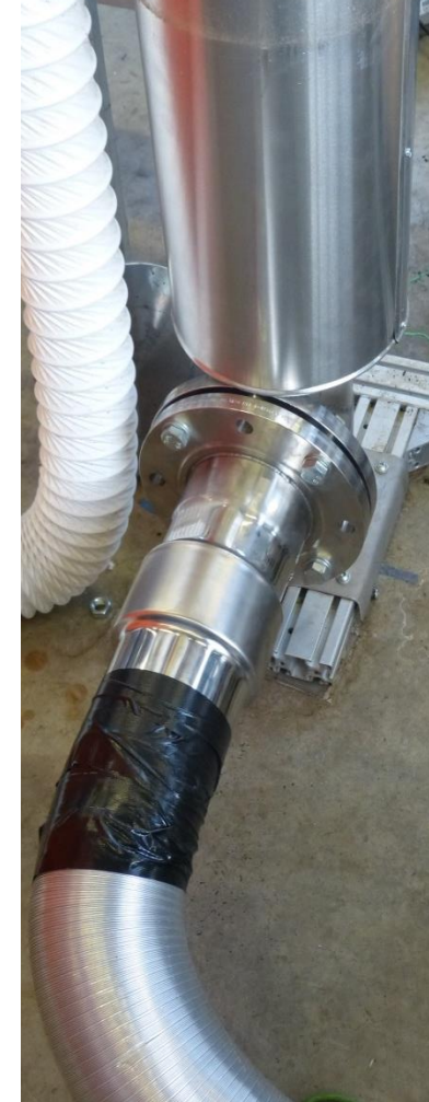
Connection to the chimney
