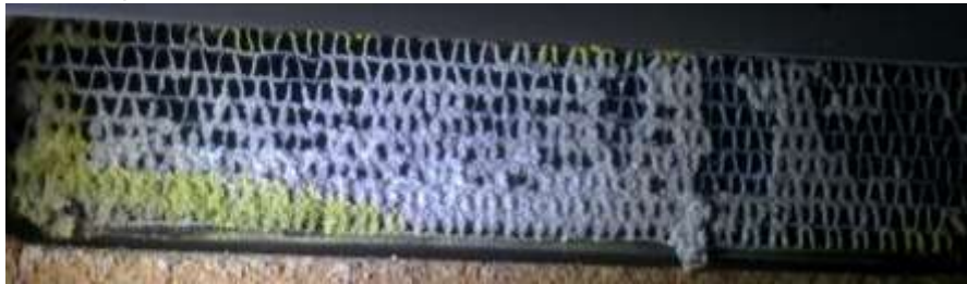
Catalyst after 2 weeks of operation (view at inlet)
