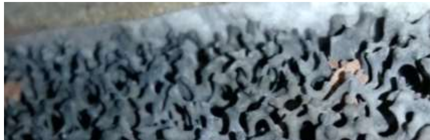
Foam ceramic after manual cleaning after 2 weeks of operation (view at inlet)
