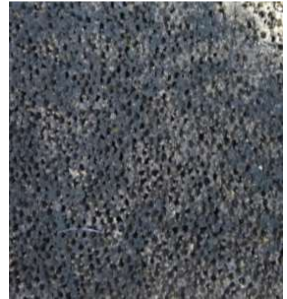
Foam ceramic after 2 heating seasons Approx. 550 batches (Filter had been washed after 1 st heating season)
