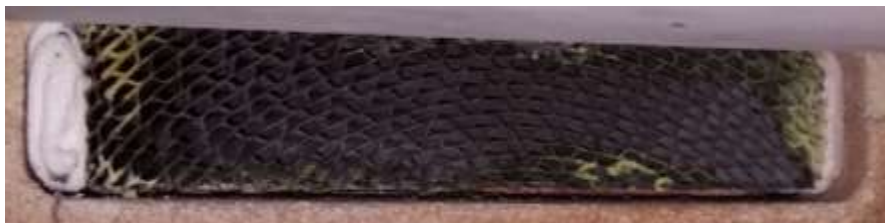
Catalyst after manual cleaning after 2 weeks of operation (view at inlet)
